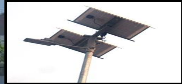
Solar Lighting System
