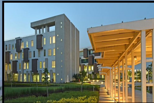
EE Internal & External lighting System
