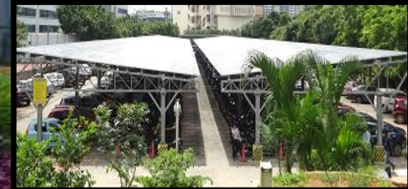
Solar Parking System
